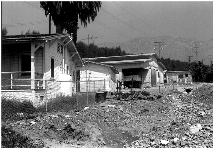
Description of Photo: (View, date, accession #) shed, barn (View toward north). Photo No: 7-13, 3/10/98
