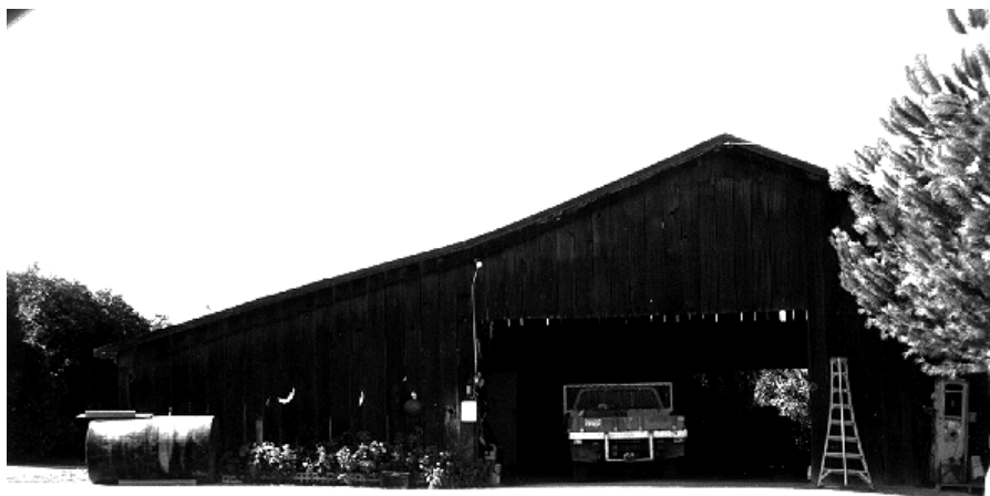
Description of Photo: (View, date, accession #) barn (View toward west). Photo No: 14-15, 11/6/98
