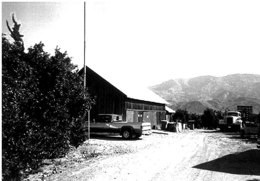
Description of Photo: (View, date, accession #) barn (View toward south). Photo No: 14-24, 11/6/98
