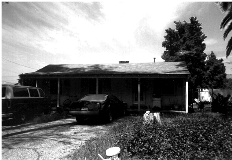
Description of Photo: (View, date, accession #) second residence (View toward west). Photo No: 5-12, 5/22/98
