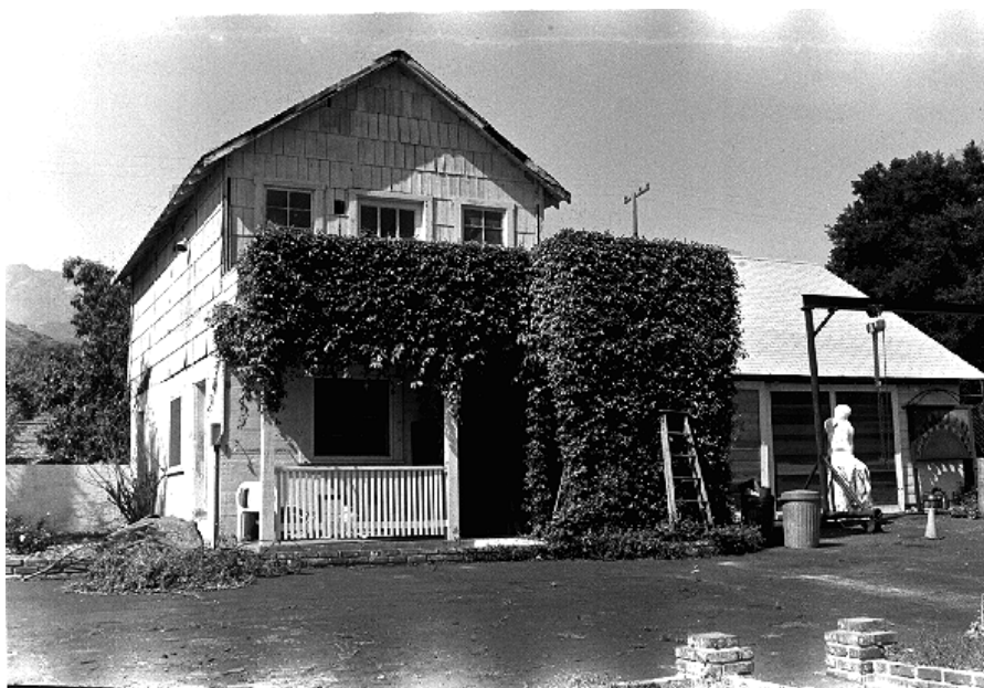
Description of Photo: (View, date, accession #) workshop/barn (View toward north). Photo No: 9-17, 4/22/98
