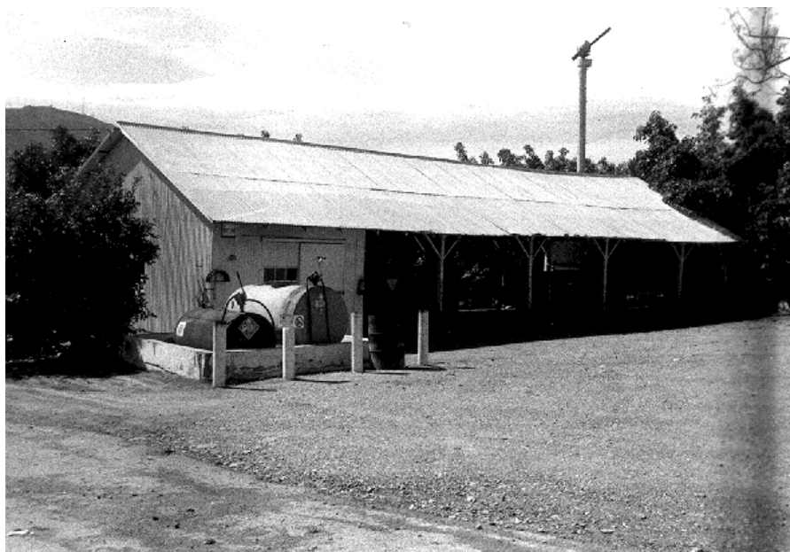
Description of Photo: (View, date, accession #) equipment shed (View toward southwest). Photo No: 8-9, 3/8/98
