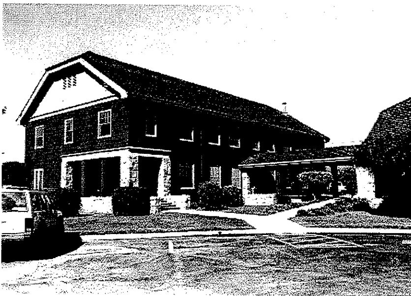
Description of Photo: (View, date, accession #) Bunkhouse, western wing, southeastern elevation.
