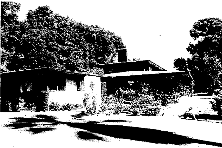
Description of Photo: (View, date, accession #) second house, southeast elevation, 9/01/95, #1629
