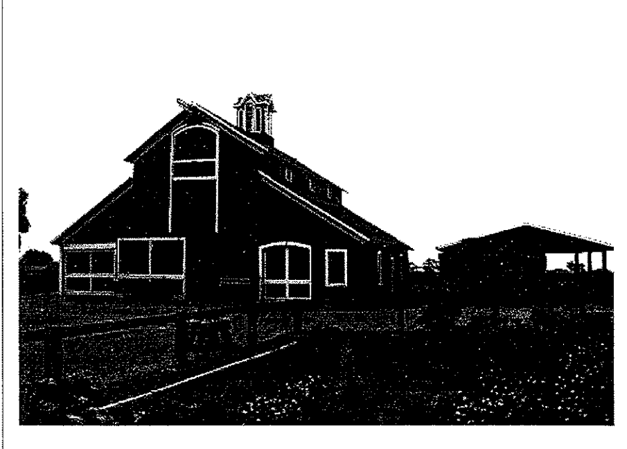
Description of Photo: (View, date, accession #) Barn, north elevation, 8/03/89, #2113
