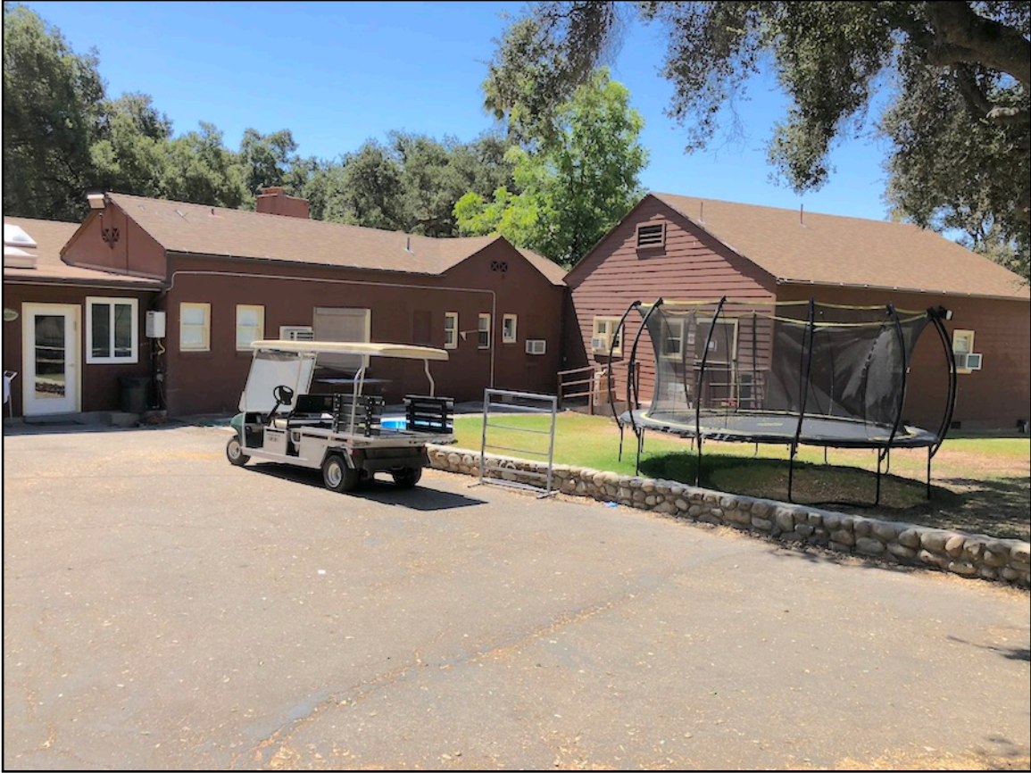
Photo 3. Preschool/Laundry, viewed from northeast. [6-30-2018]
