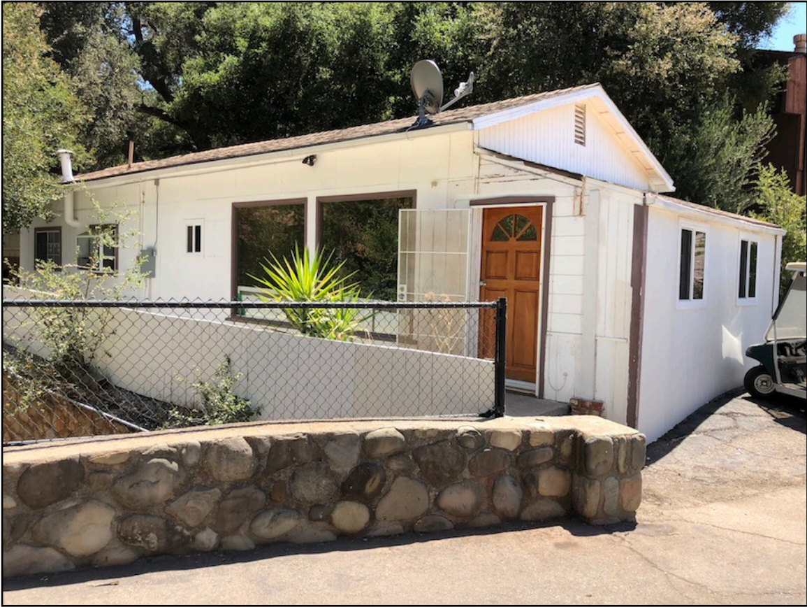
Photo 15. Staff Housing, viewed from west. [6-30-18]
