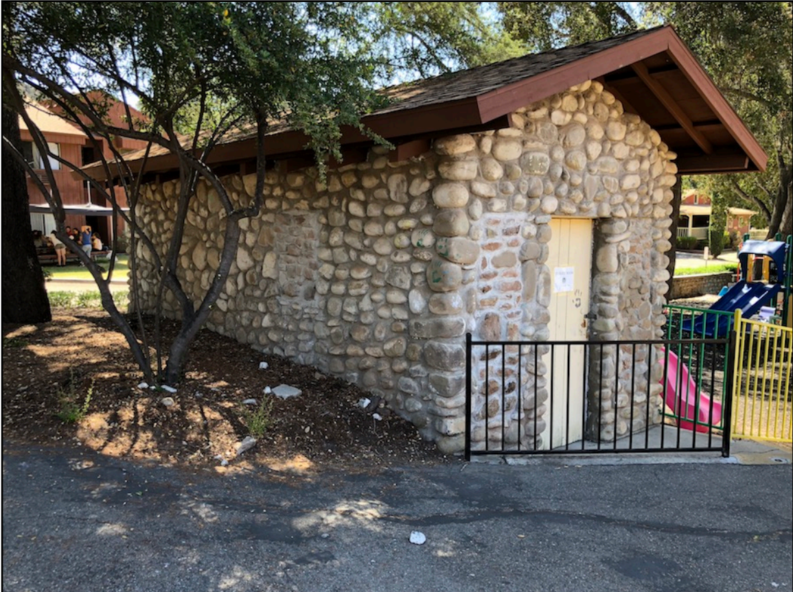
Photo 4. Cold Room, viewed from northwest. [6-30-2018].
