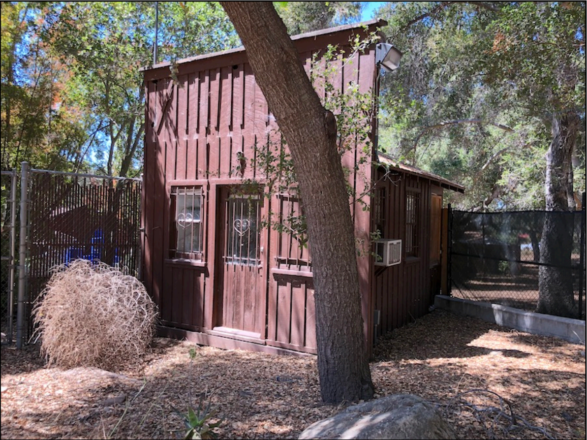
Photo 12. Entry Building, viewed from north. [6-30-18]
