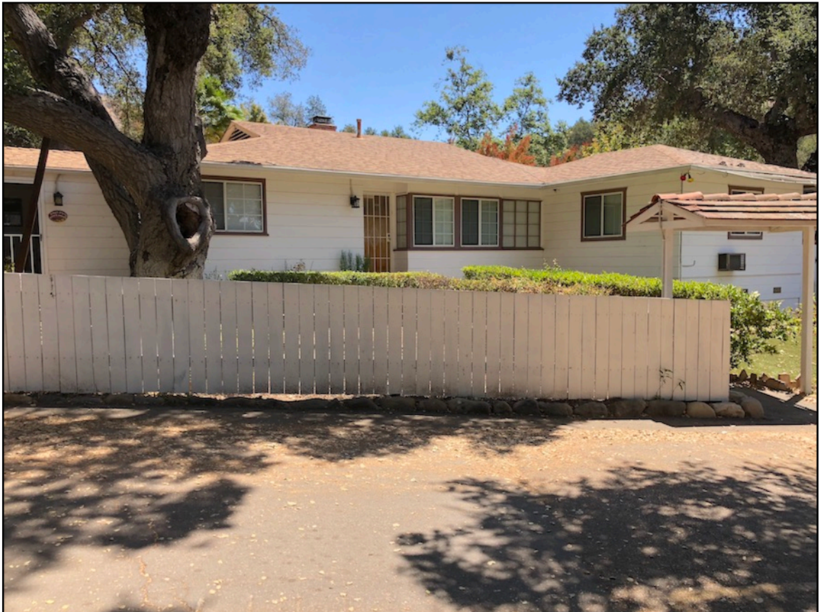
Photo 10. Manager's House, viewed from west. [6-30-18]
