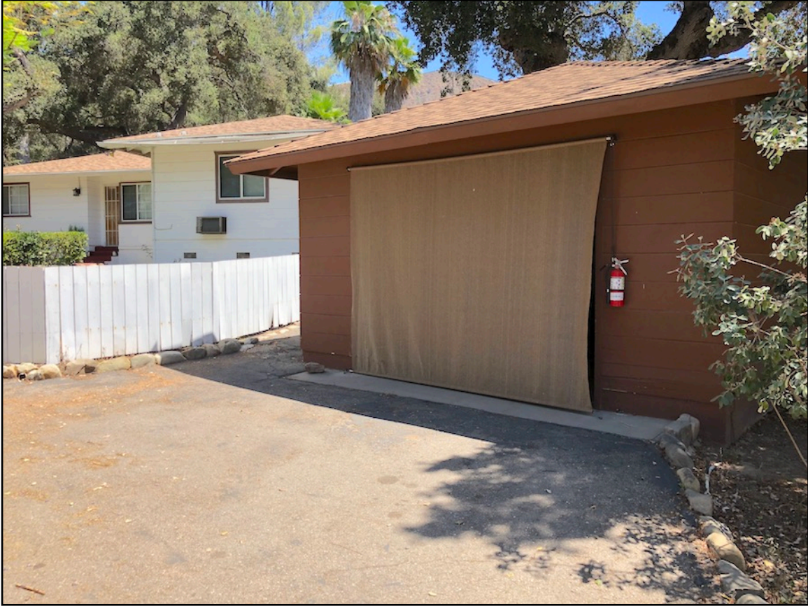
Photo 11. Manager's House and garage, viewed from southwest. [6-30-18]
