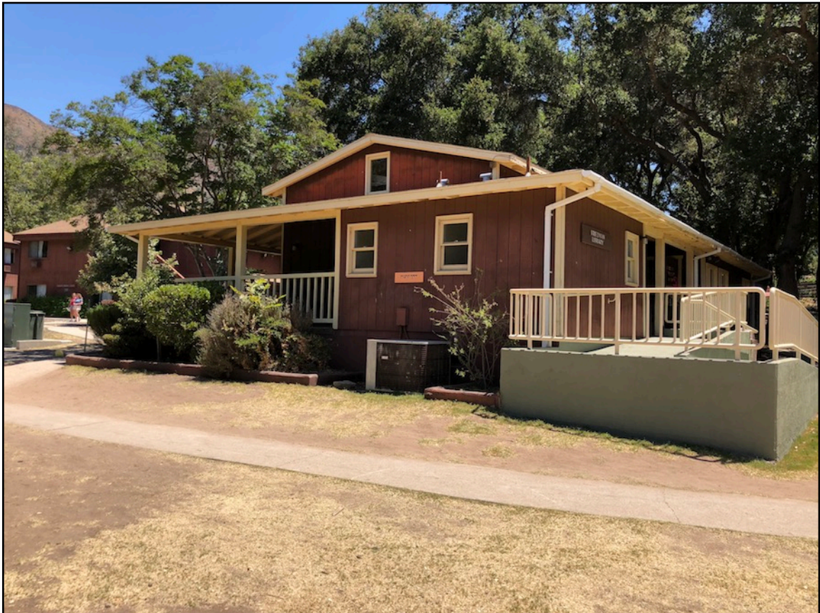
Photo 8. Friedman Library, viewed from southwest. [6-30-18]
