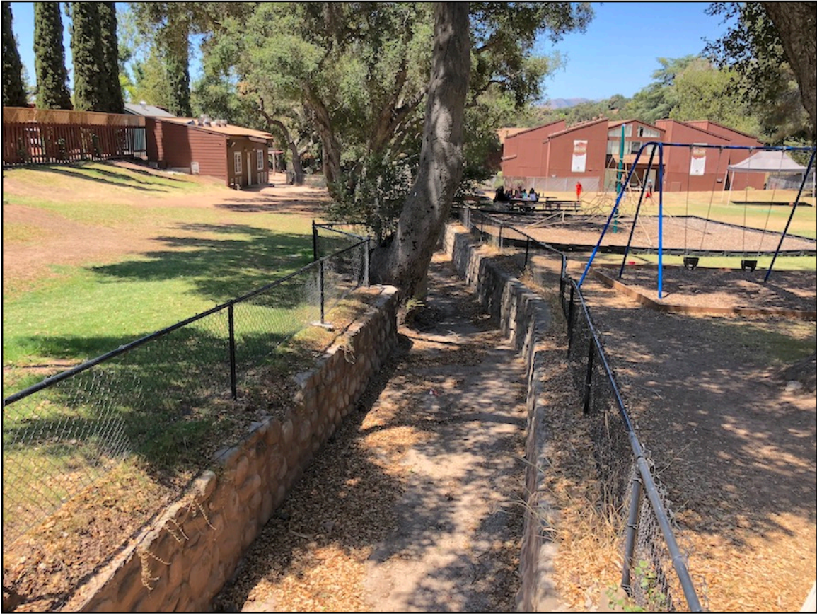
Photo 19. Stone-lined creek channel. [6-30-18]
