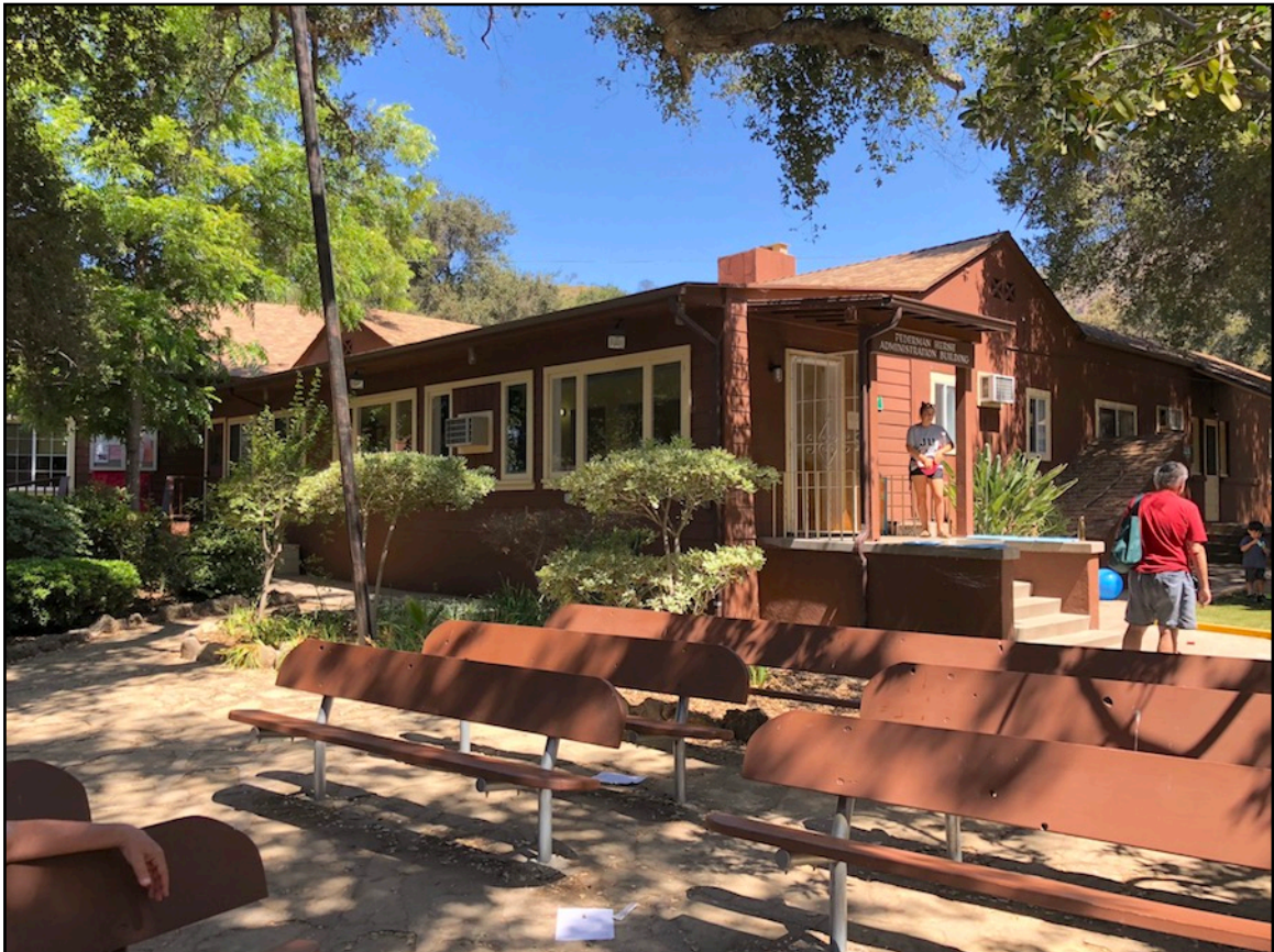
Photo 2. Administration Building/Preschool, viewed from southeast. [6-30-2018]
