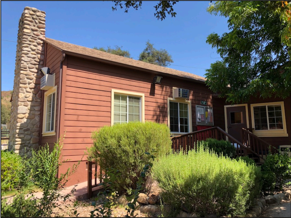
Photo 1. Administration Building, southern wing, viewed from south. [6-30-2018]
