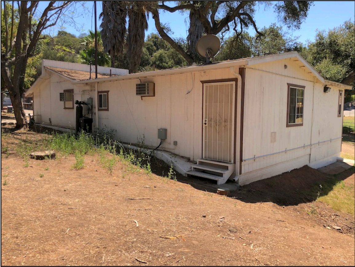
Photo 9. Caretaker's House, viewed from northwest. [6-30-18]
