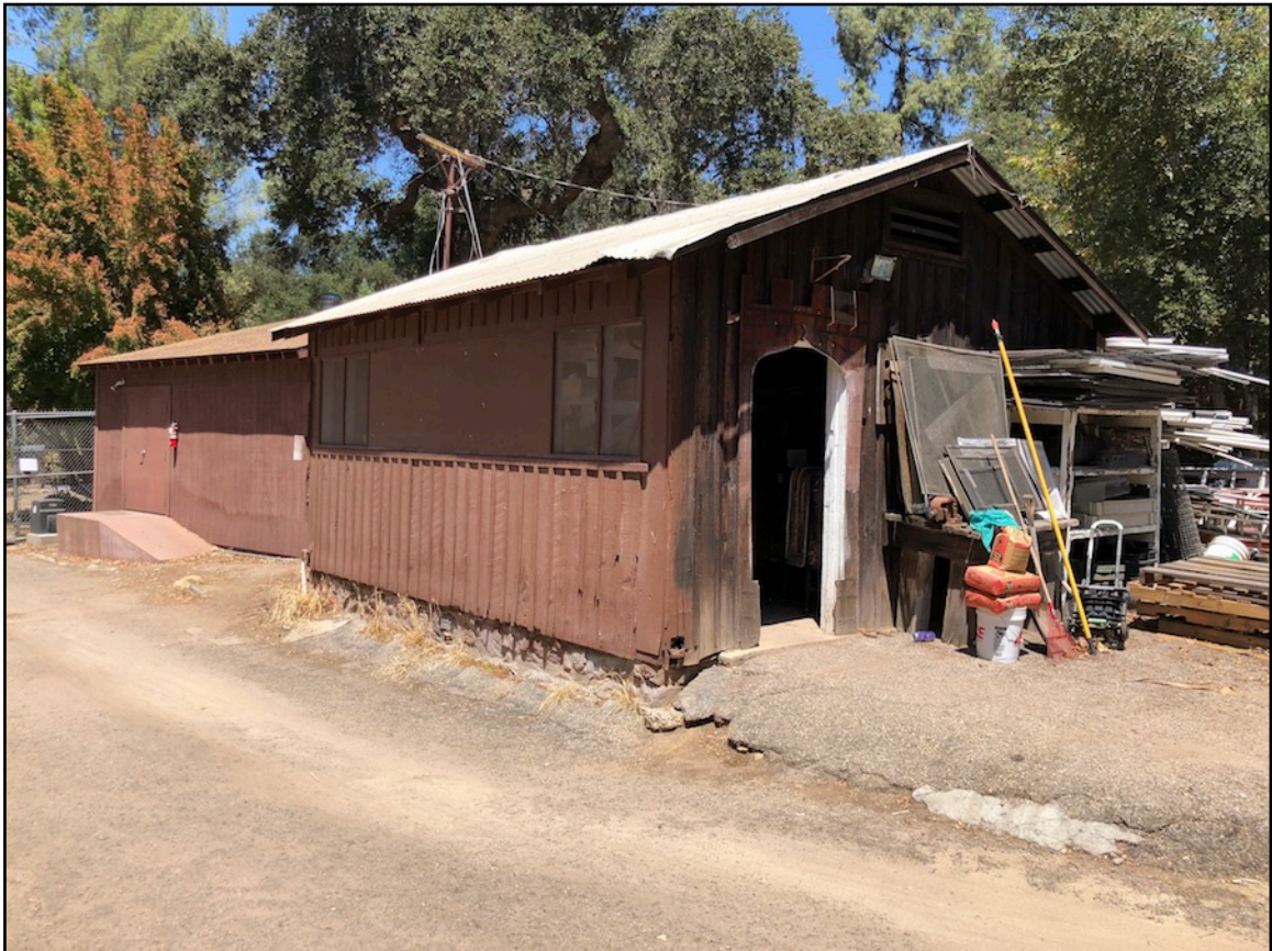
Photo 14. Photo 13. Maintenance Yard. [6-30-18]
