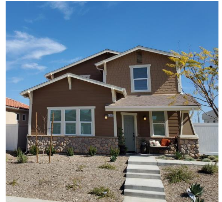
Picture location: New housing, Piru
