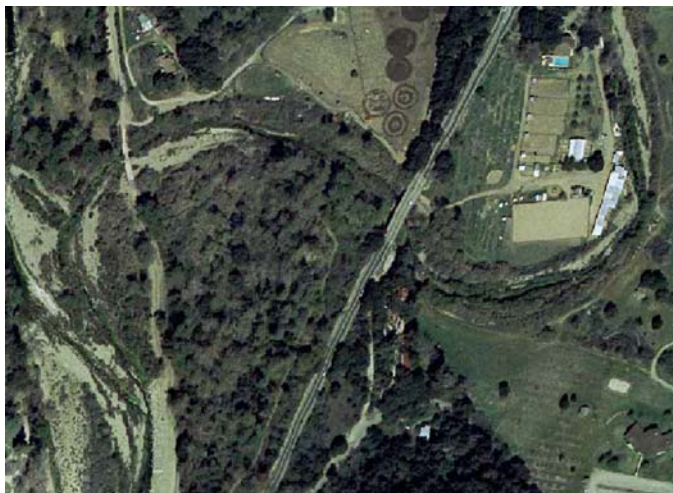
Figure 55. San Antonio Creek passing under Highway 33 to join the Ventura River.
