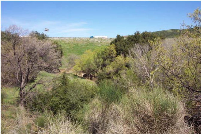
Figure 52. Spectacular riparian forest and oval concrete culvert under I-5 at Big Oak Flat (center).
