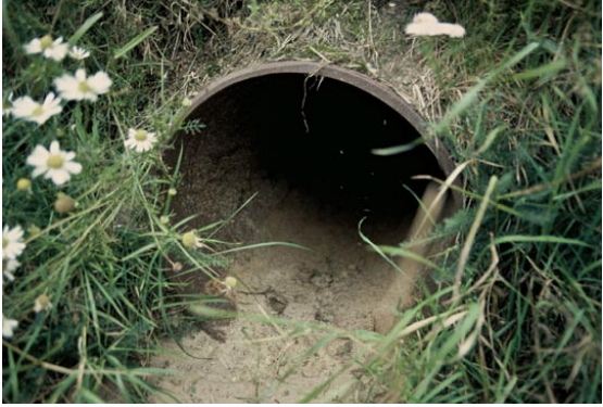
Figure 42. Pipe culvert designed to accommodate small mammals.
