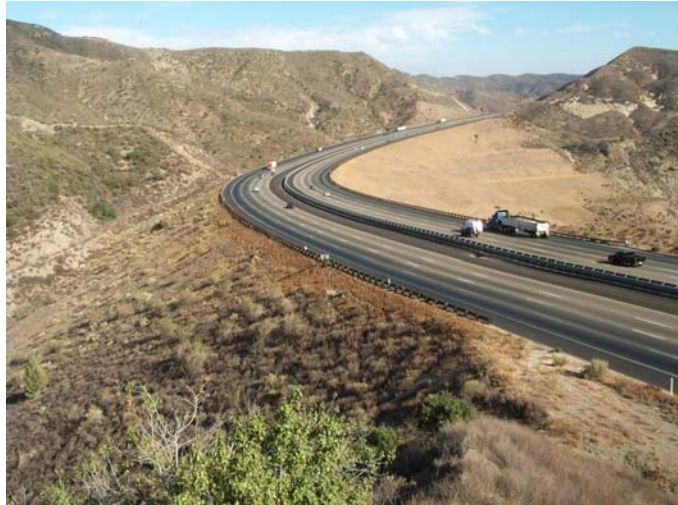
Figure 48. Potential site for vegetated landbridge on I-5 on the east ridge of Cherry Canyon. Currently, deer and other species are crossing at grade and the topography would permit construction of a vegetated overpass here.
