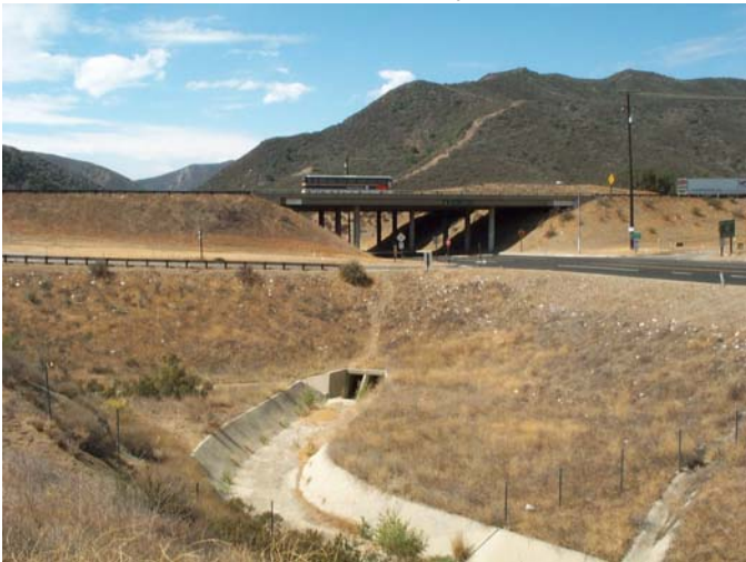
Figure 54. Templin Highway underpass.
