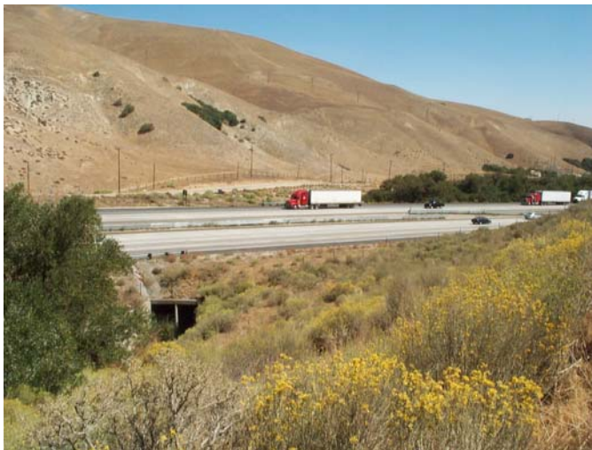
Figure 44. Gorman Creek flows through a series of concrete box culverts.
