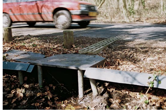
Figure 43. Amphibian tunnels allow light and moisture into the structure.
