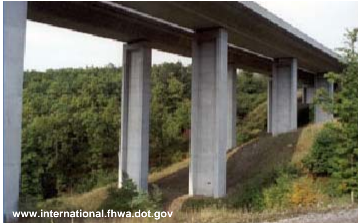
Figure 40. A viaduct in Slovenia built to accommodate wildlife, hydrology, and human connectivity.
