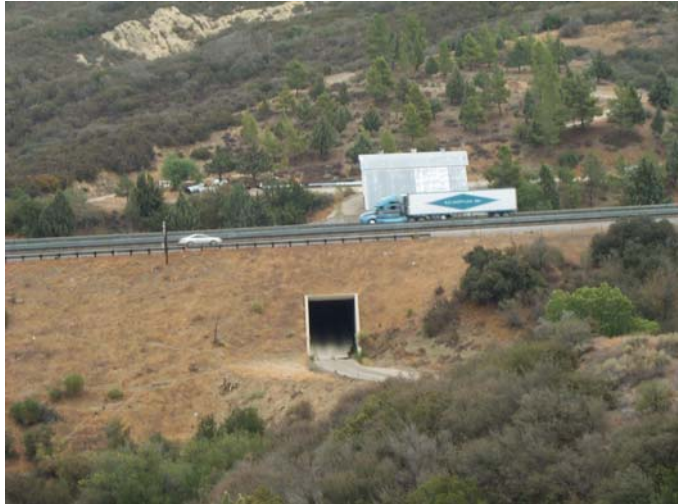
Figure 50. Box culvert for Forest Service Road 6N43 under I-5.
