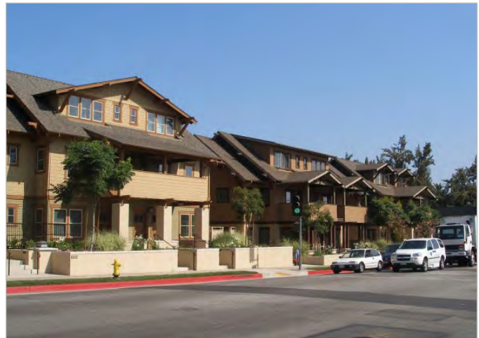
The scale of multi-family buildings can be reduced by placing the third story in the attic space.
