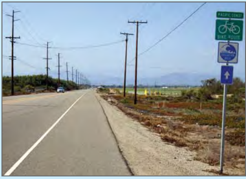
Harbor Boulevard includes a Class 2 Bike Lane
