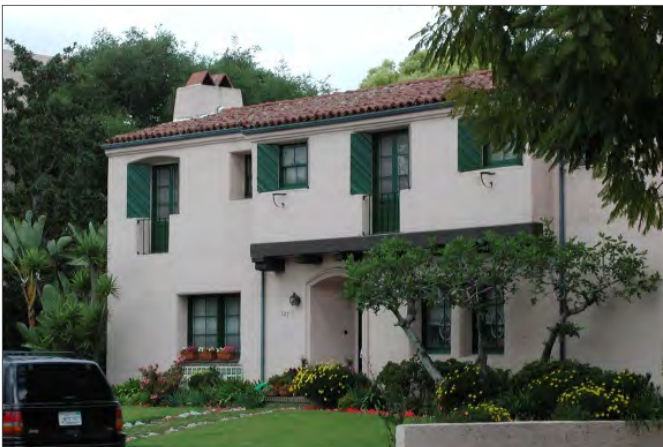
Example of a residential building that uses an overhanging room to break up its front façade.
