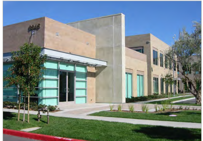
Image 6.15. Trees, landscaping, and decorative paving around building entry highlights access to the development.
