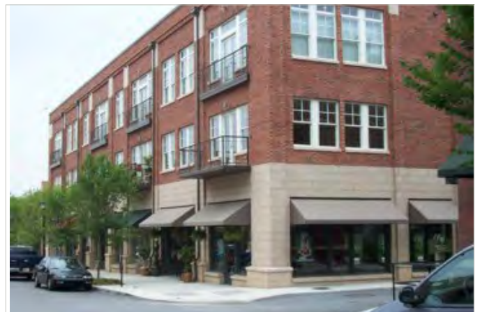
Example of a mixed-use building that employs pilasters to divide its façade into vertical bays.
