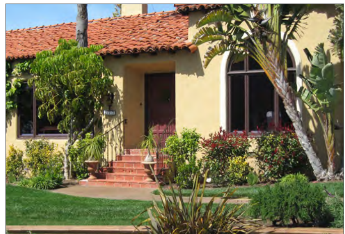
Stoop Example - stairs, landing, and landscape area.
