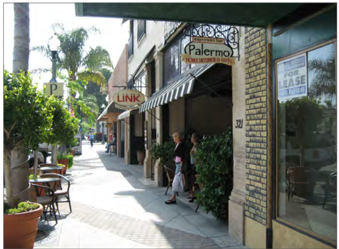
Shopfront Example - large glazing area of display windows, tile bulkhead under windows, glass door, clerestory and shade awning.
