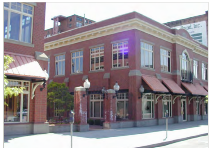
Image 6.4. A “Main Street” commercial building, with simple massing, with access from the street.
