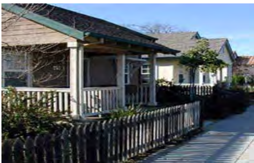
Landscaping serves as a focal point and buffers residences from parking areas.
