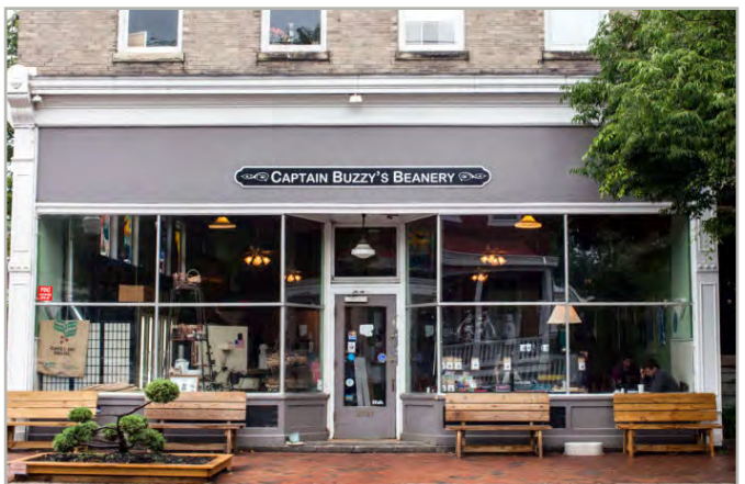
Shopfront Example - large glazing area of display windows, and recessed storefront entry with glass door.
