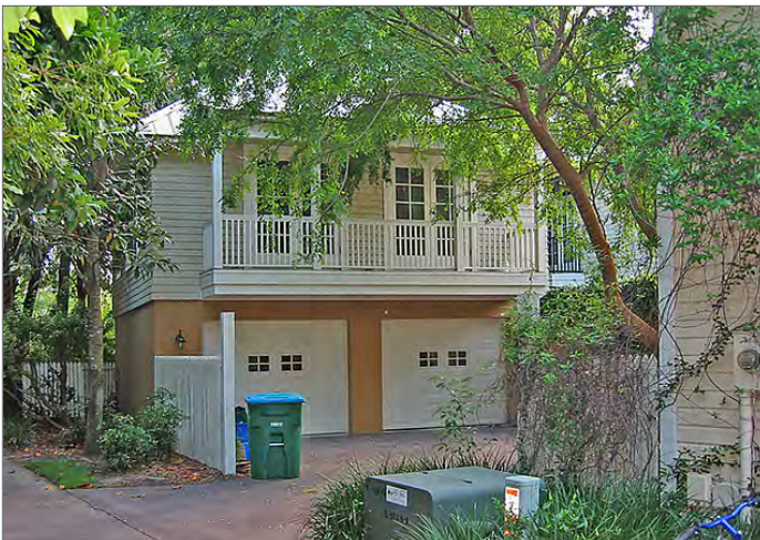
Illustrative Photo of a ground-floor non-habitable garage, configured with a habitable accessory unit above it with no internal access and detached from the principal dwelling.
