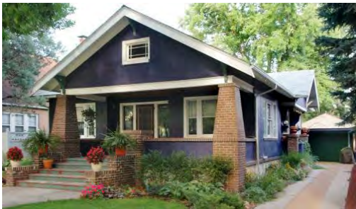
Placing detached garages in the back of the site creates a more desirable scene.
