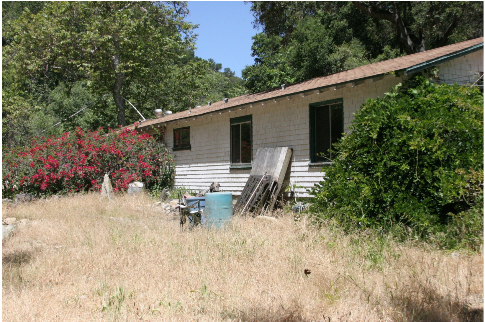
Photo #1b Bathhouse, ca. 1920s Matilija Hot Springs Site plan #2 (Brian Fortune, FVP Images, June 6, 2012)
