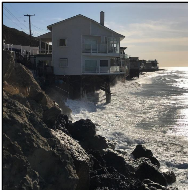
Photo 3-5: Residence constructed on pilings during a king tide on December 3, 2017.
