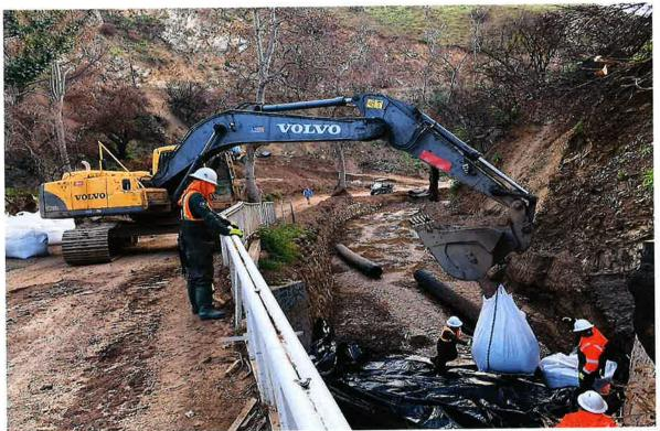
Photograph 5. Constructing Diversion 1. Note excavator lowering super sacks into the channel (facing south) (4/1/19)
