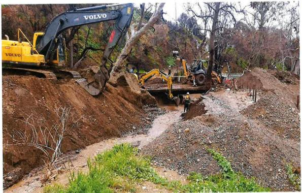
**Photograph 3.** View of equipment staged outside of the creek and removing sediment from the creek (facing south) (3/5/19).
