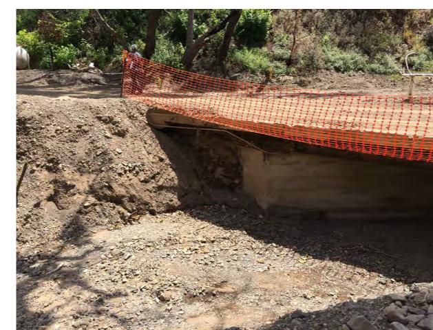
ADD ROCK PROTECTION AT BRIDGE ABUTMENT PER DETAIL "B", SHEET 3.
