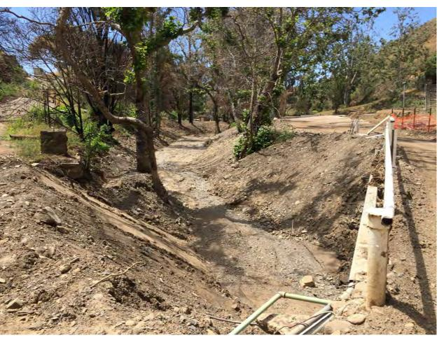
BANK STABILIZATION AREAS; 460± SF & 480± SF RECONSTRUCT BANKS PER DETAIL "A", SHEET 3.
