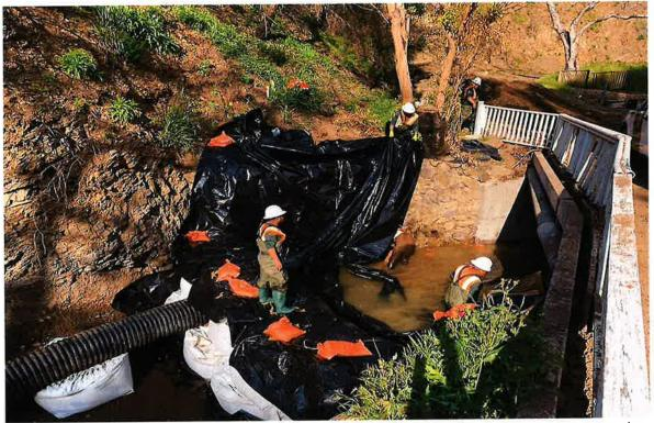
Photograph 7. Completing the temporary, upstream coffer dam of Diversion 1. Note visqueen around super sacks to avoid sedimentation within the creek (4/2/19).
