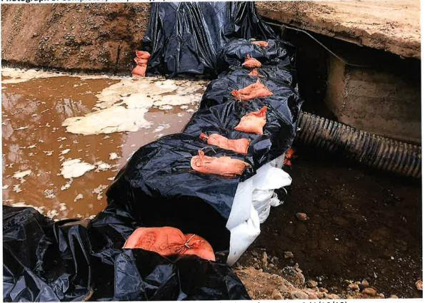
Photograph 10. Completed, temporary, upstream coffer dam of Diversion 3 (4/16/19).
