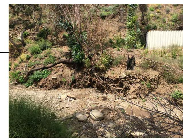
BANK STABILIZATION AREA; 30± SF RECONSTRUCT BANK WITH 3' HIGH 1'-2' DIAMETER ROCKS TO PROTECT SLOPE UNDER TREE.
