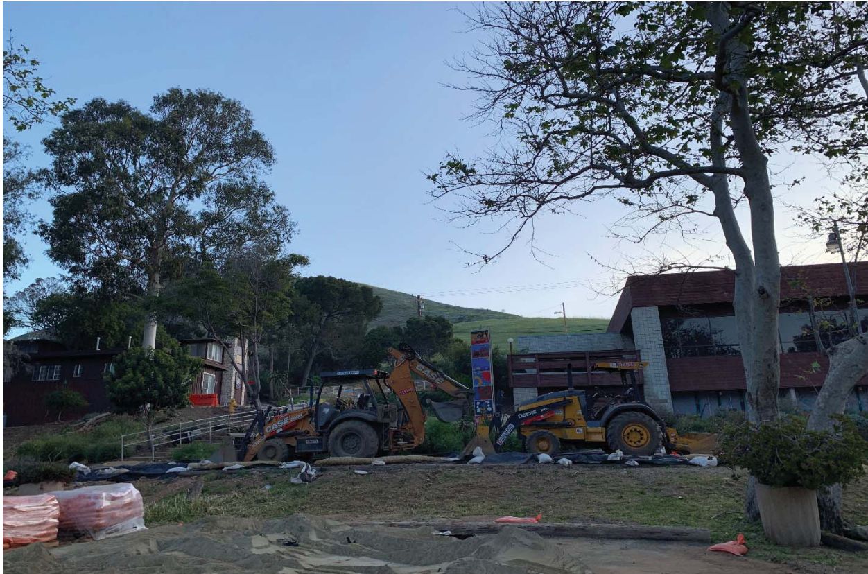
Photograph 6. Visqueen and straw wattles around equipment in the staging area (4/2/19).
