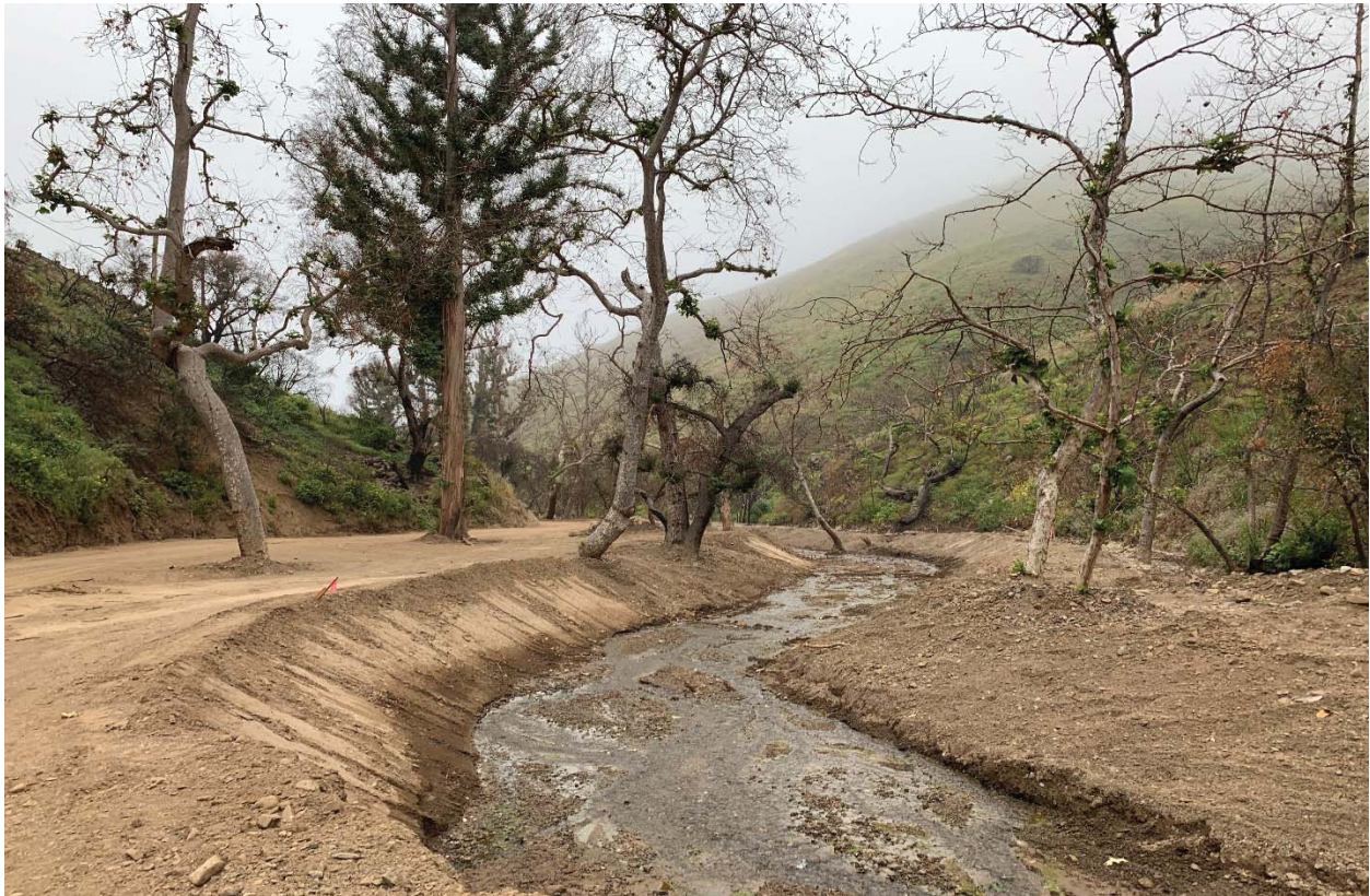
Photograph 12. View of creek within Diversion 1 location, post-diversion removal (facing south) (4/25/19).
