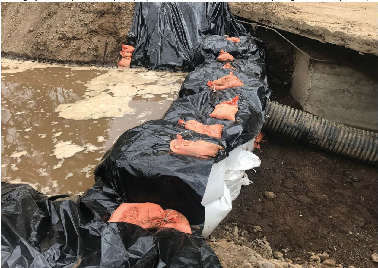
Photograph 10. Completed, temporary, upstream coffer dam of Diversion 3 (4/16/19).
