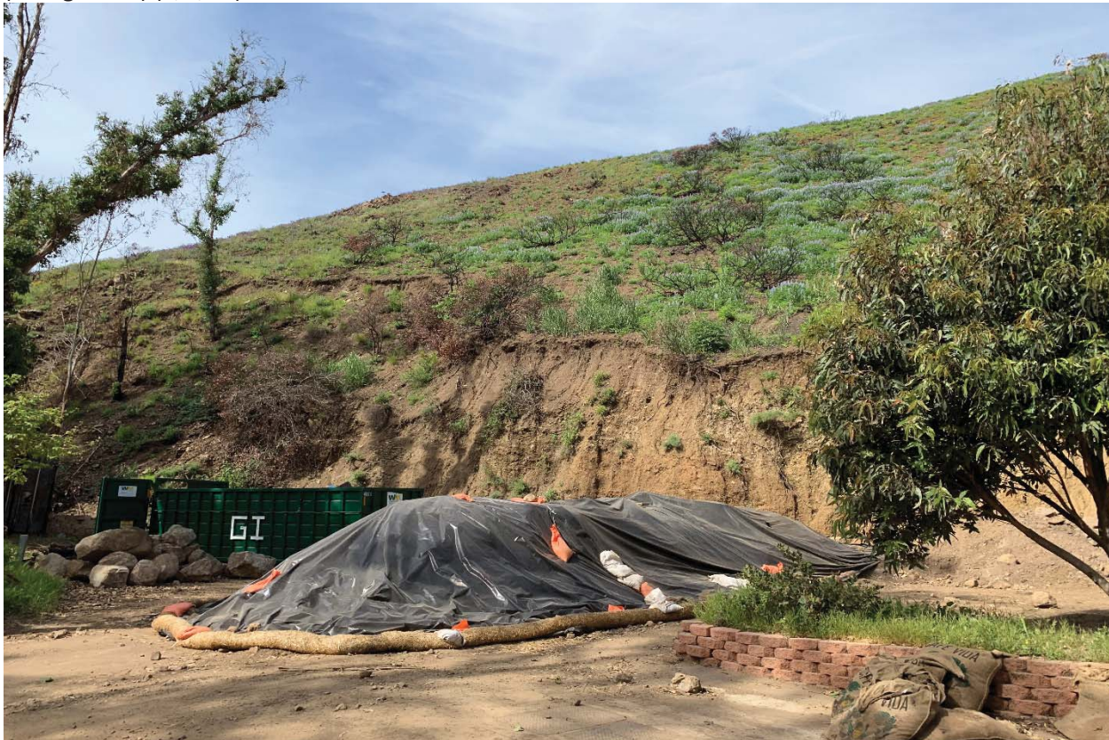
Photograph 4. Visqueen and straw wattles placed around the stockpiles (3/19/19).
