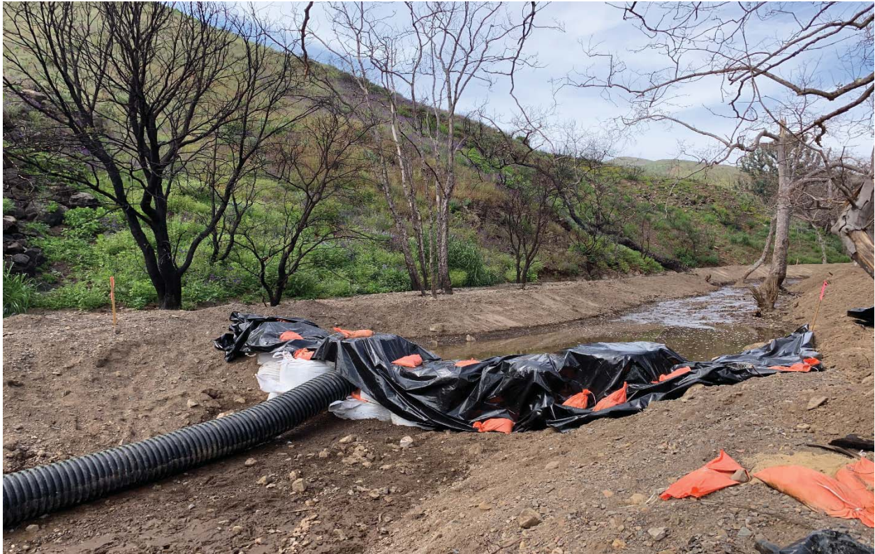
Photograph 9. Completed, temporary, upstream coffer dam of Diversion 2 (facing northwest) (4/8/19).
