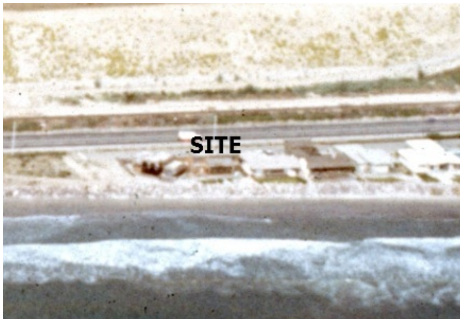
Photograph 2. Subject site and shoreline in 1972. Note that the continuous revetment fronting the properties in the site area.
