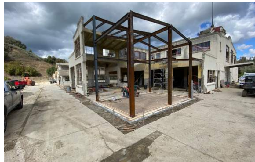
Re-built Steel Structure
