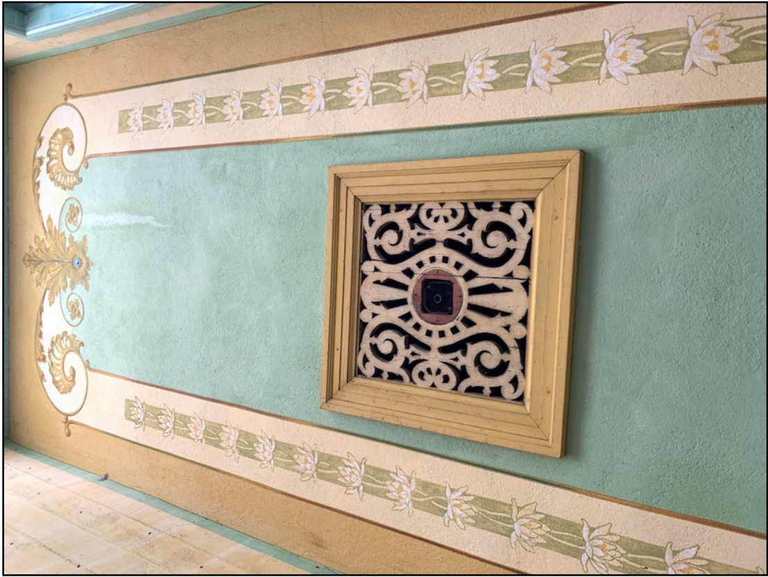
Photo 9. Creamery interior ceiling stenciling detail. [10-16-19]
