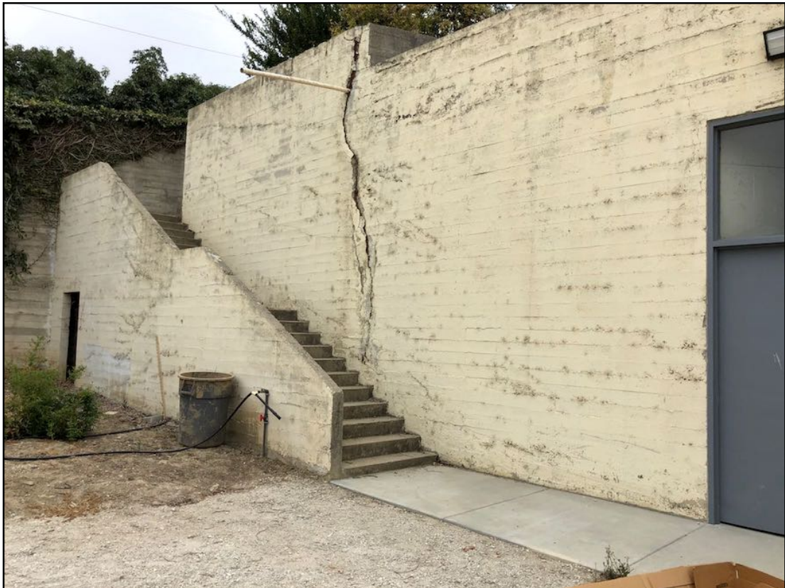
Photo 14. Dormitory basement, southern elevation. [9-27-19]
