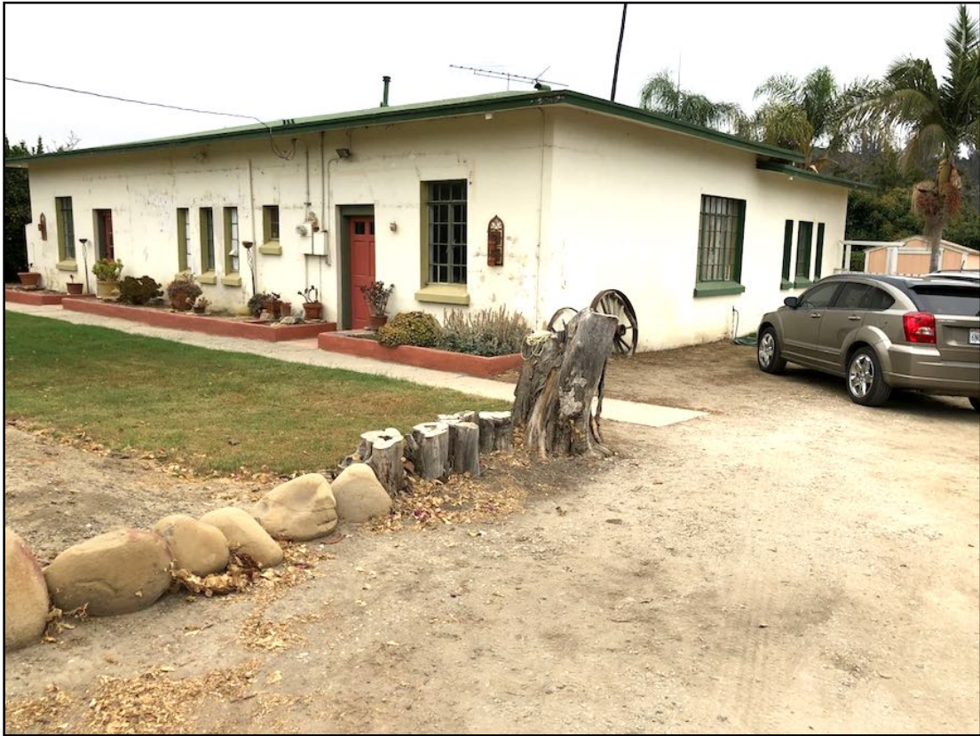
Photo 13. Office, western and southern elevations. [9-27-19]
