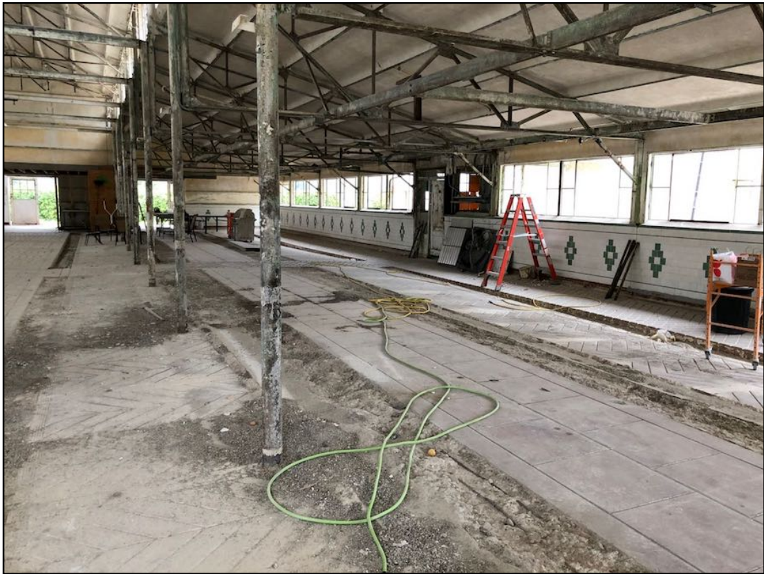
Photo 4. Interior of Milking Barn with wall tile and concrete details. [9-27-19]
