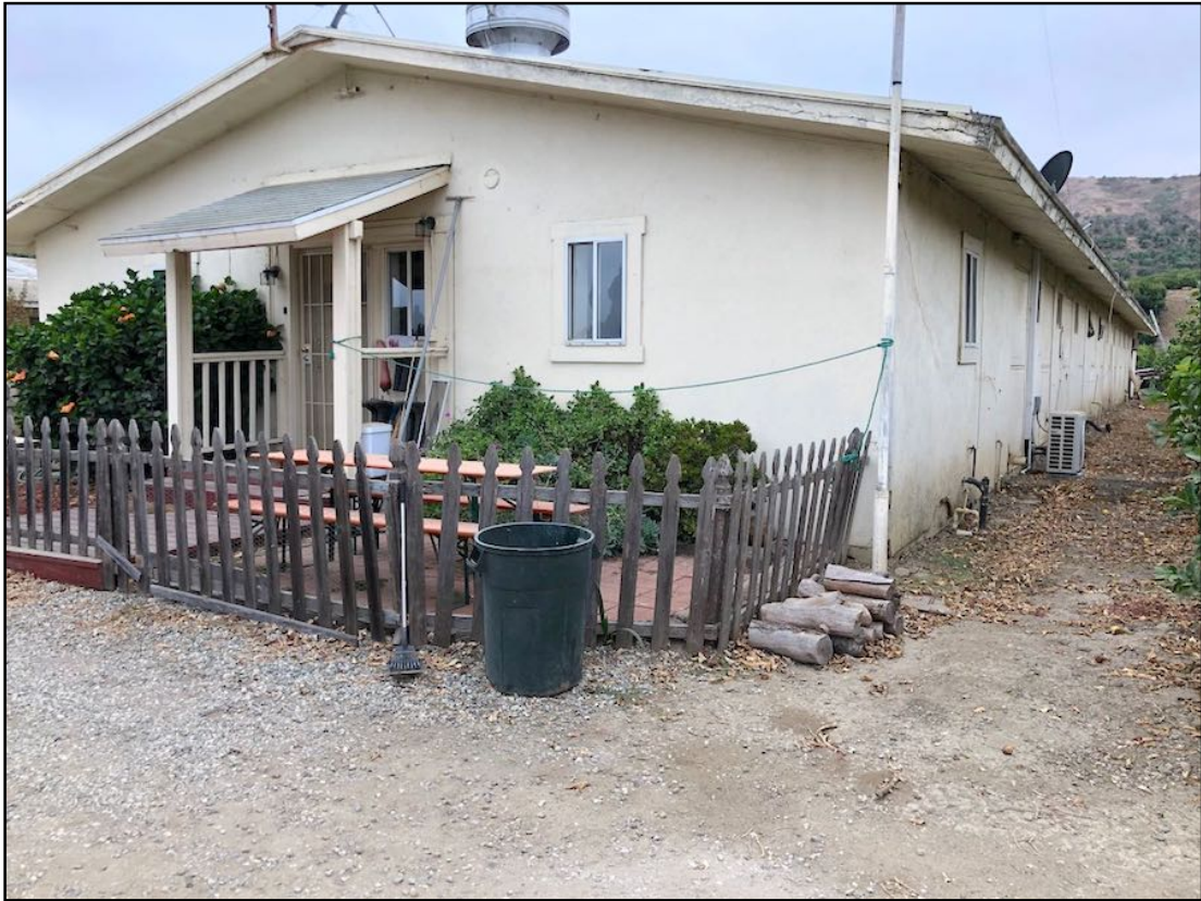
Photo 11. Cow Barn (Building 2), northern and eastern elevations, altered door and window openings with porch addition. [9-27-19]
