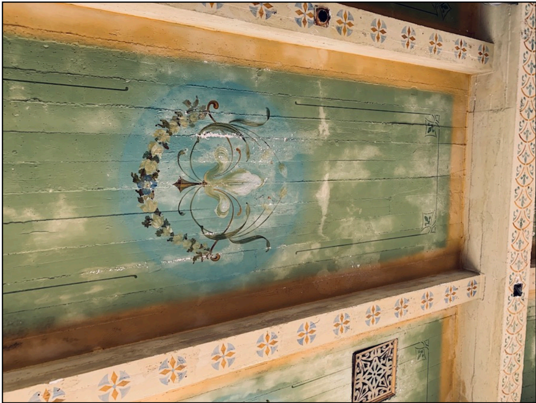
Photo 8. Creamery interior ceiling stenciling detail. [10-16-19]
