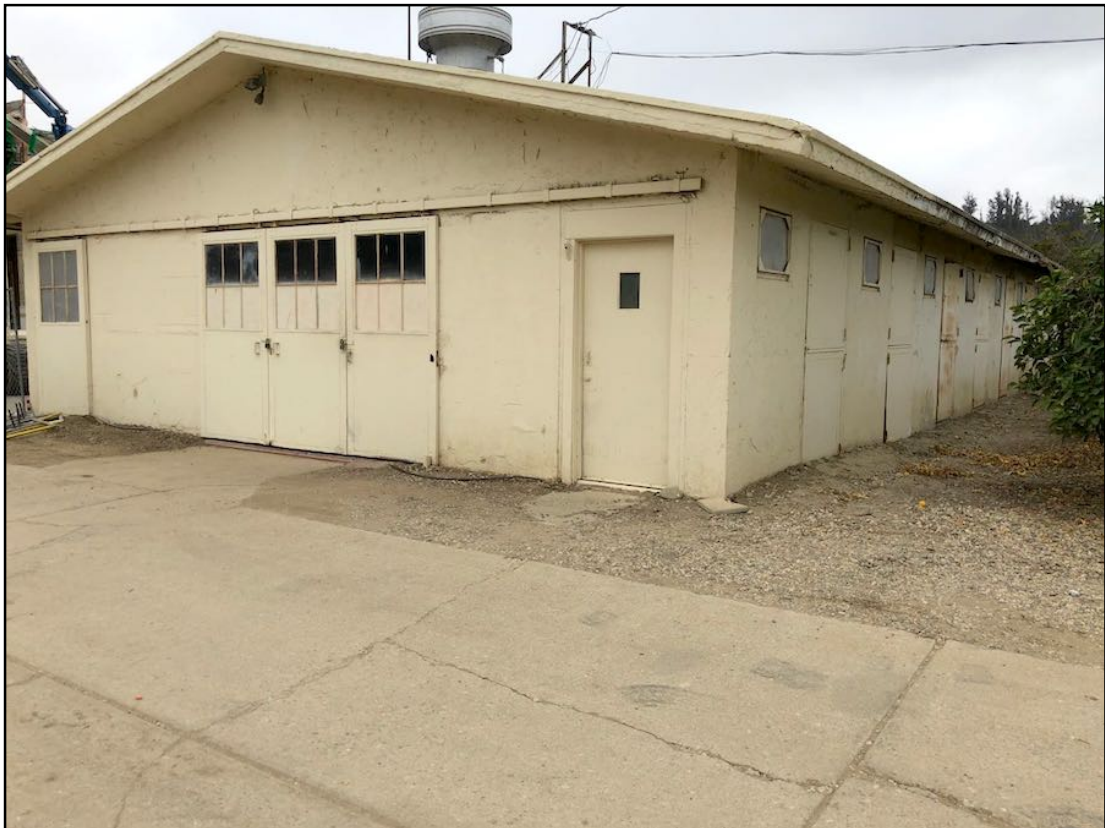
Photo 10. Cow Barn (Building 3), southern and western elevations. [9-27-19]
