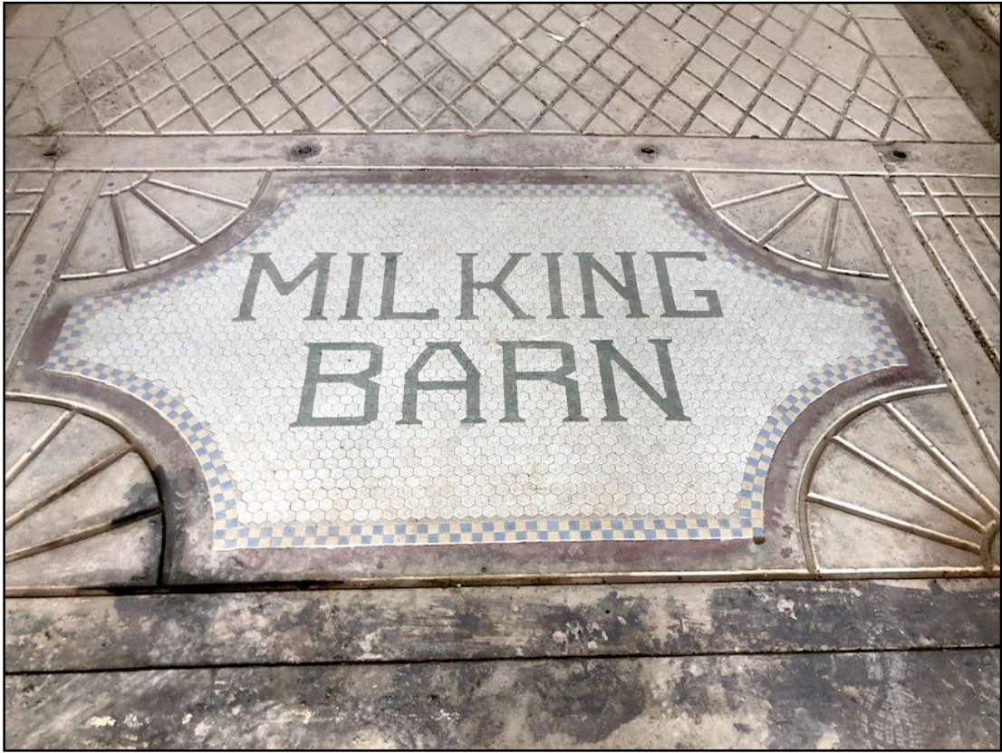
Photo 5. Milking Barn interior floor tile and concrete detail. [9-27-19]
