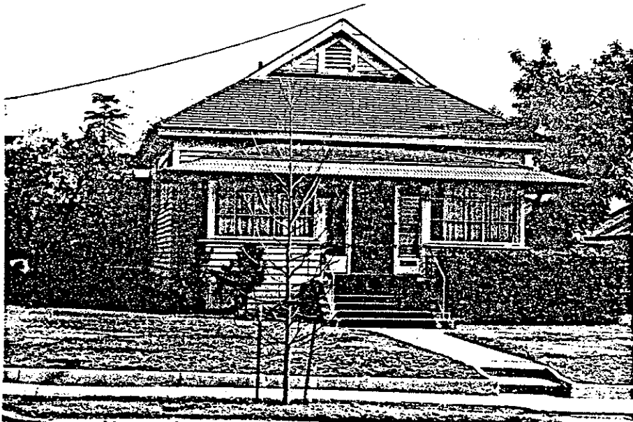
309 North Mill Street
