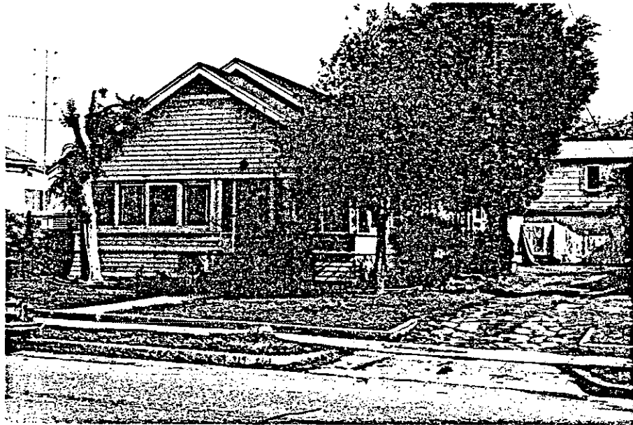
315 North Mill Street
