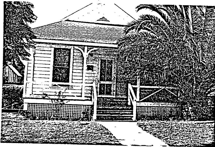
324 North Mill Street
