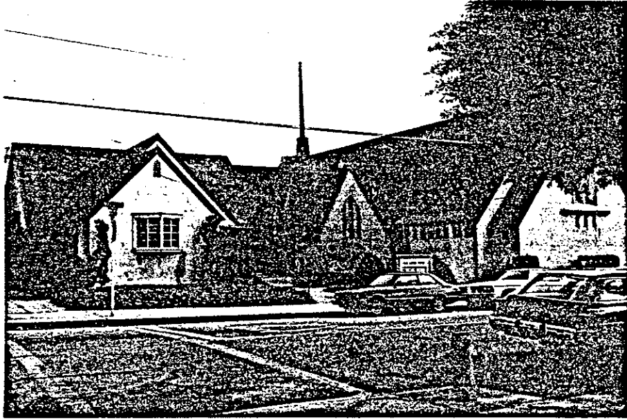
241 North Mill Street
