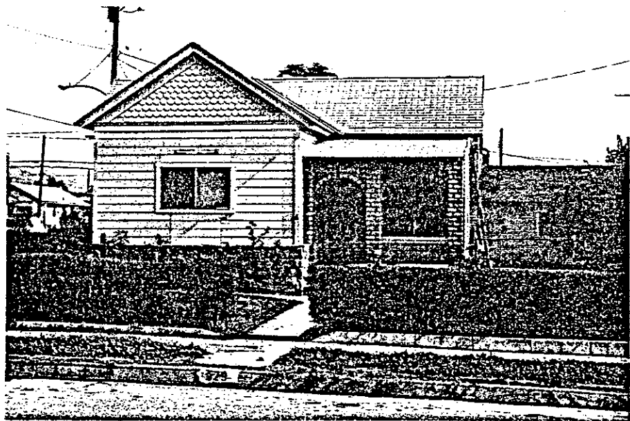
329 North Mill Street
