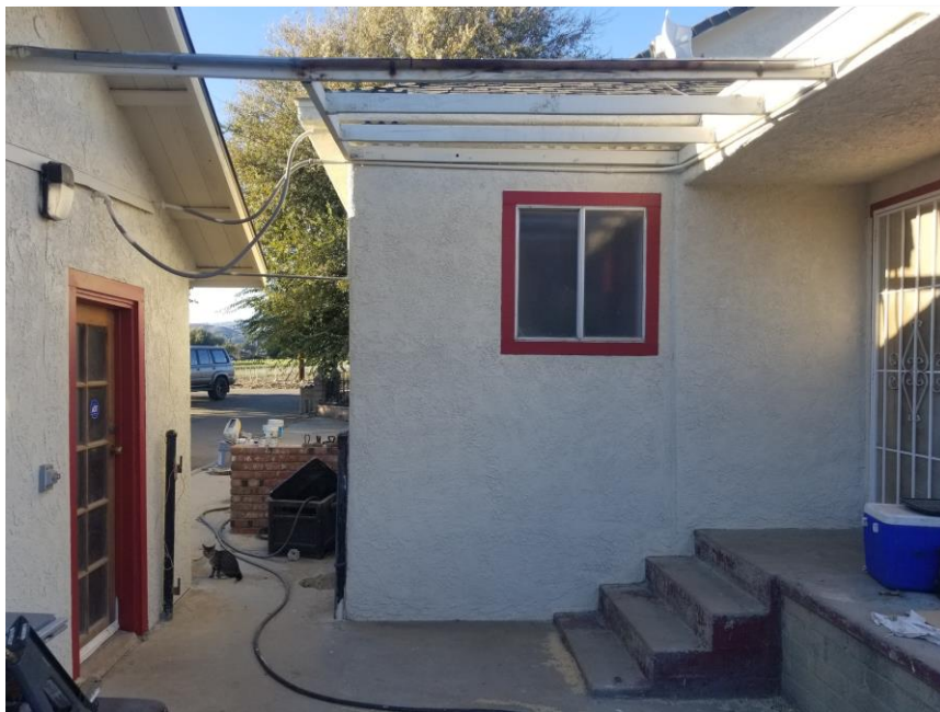
Figure 8 – View of Residence, Looking North
