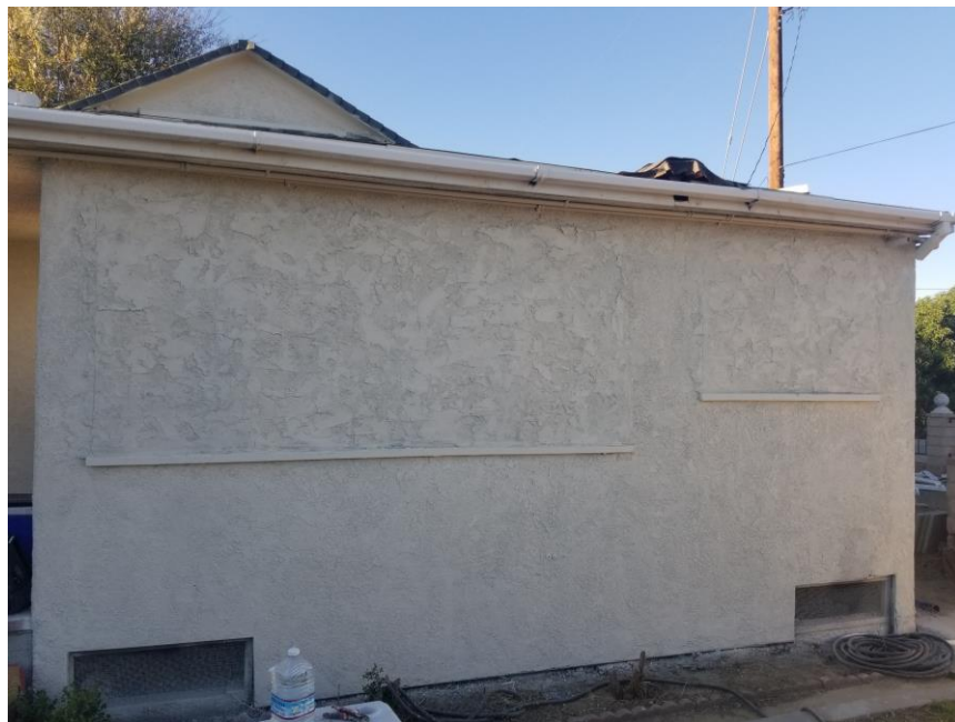
Figure 6 – View of Residence, Looking North
