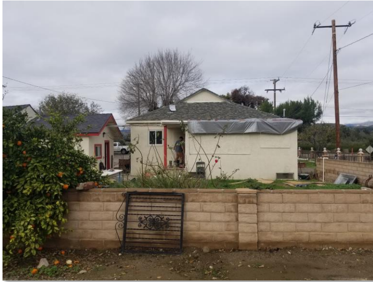
Figure 5 – View of Residence, Looking North
