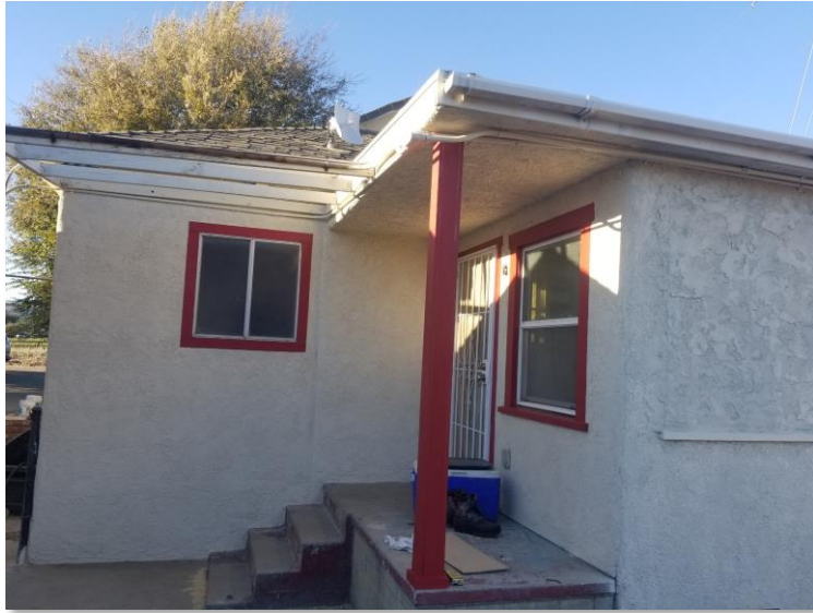
Figure 7 – View of Residence, Looking North
