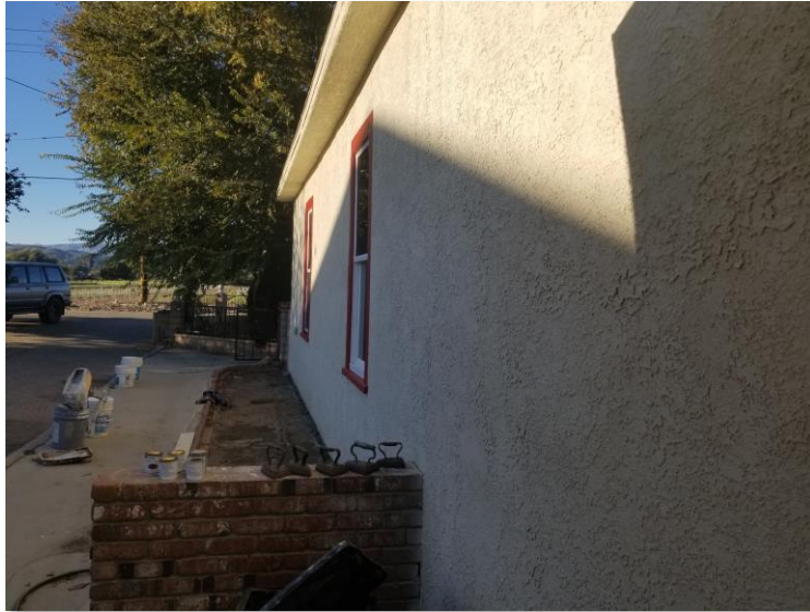
Figure 9 – View of Residence, Looking North
