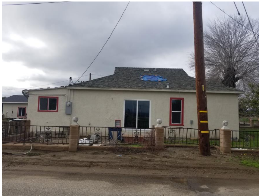
Figure 2 – View of Residence, Looking West
