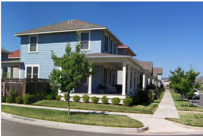
Example of a building that incorporates the same materials and finishes on both its Primary Street and Side Street façades. Its front porch also faces both streets.
