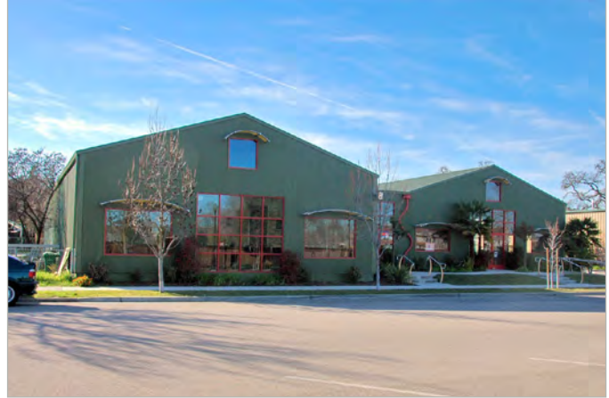
Image 6.9. An industrial building with non-reflective metal siding, appropriate only for the IND zone.
