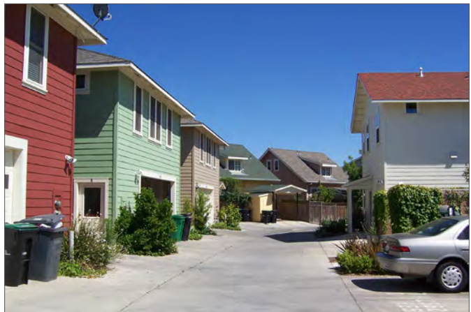
Accessory buildings have alley-facing windows.
