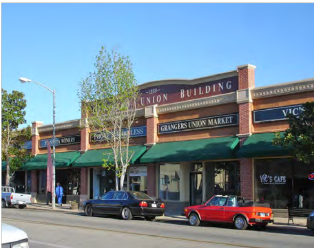
Image 6.13. A "Main Street" commercial building with a flat roof screened by parapet walls.
