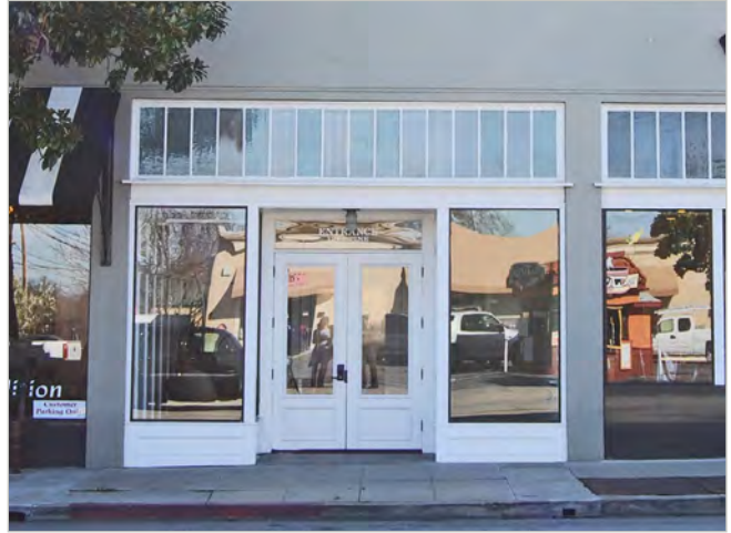
Image 6.6. A commercial shopfront oriented towards the public street, with a recessed entry door. Doors and windows across the primary shopfront are made of wood or similar materials.
