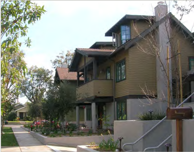
Image 6.12. Step-backs and changes in rooflines help create the illusion of smaller scale buildings, appropriate for a residential neighborhood.
