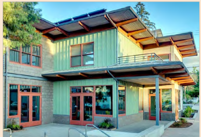
A commercial building with excessive roof breaks. The disorganized placement of rooflines and the multiple orientations of the windows, do NOT embody the intent of the guideline.
