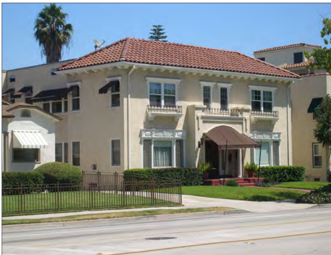
Illustrative Photo of a small apartment building.
